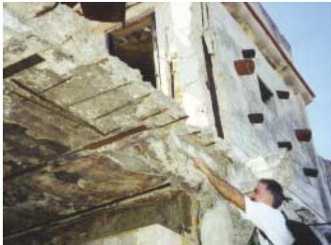
Fig. 1: Corrosion-induced damage in a concrete structure
